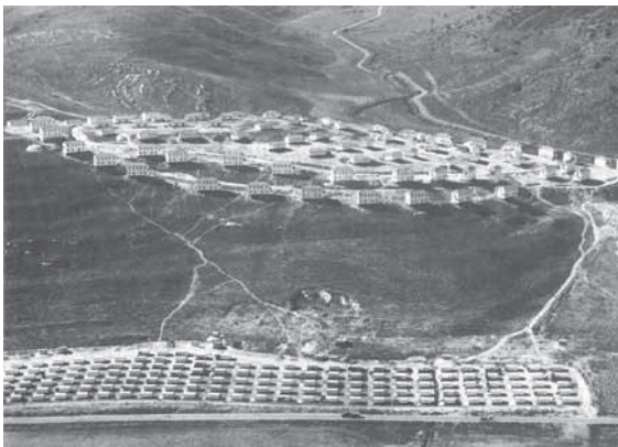
Fig. 11: A neighborhood unit in the new town of Yokne'am, being constructed by the immigrants who lived in provisional shacks along the road 19 .
